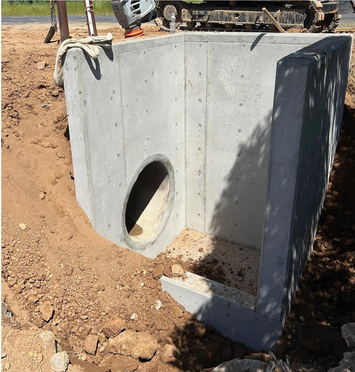
New Outfall on the East Ditch Near Brandt Road
