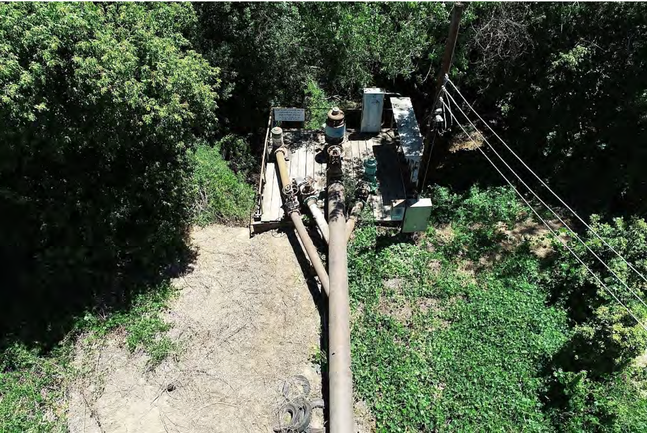
NORTH PUMP STATION
