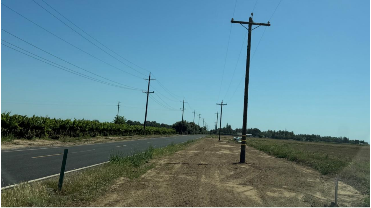
North System Pipeline re compacted
