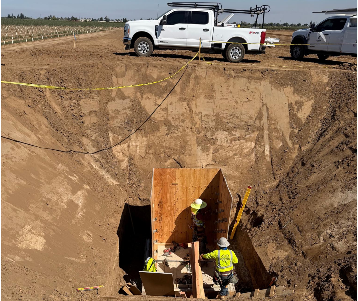
Arnaudo Framing the box that will direct water back into the South Main Pipeline at the Toe of Locust Tree Basin
