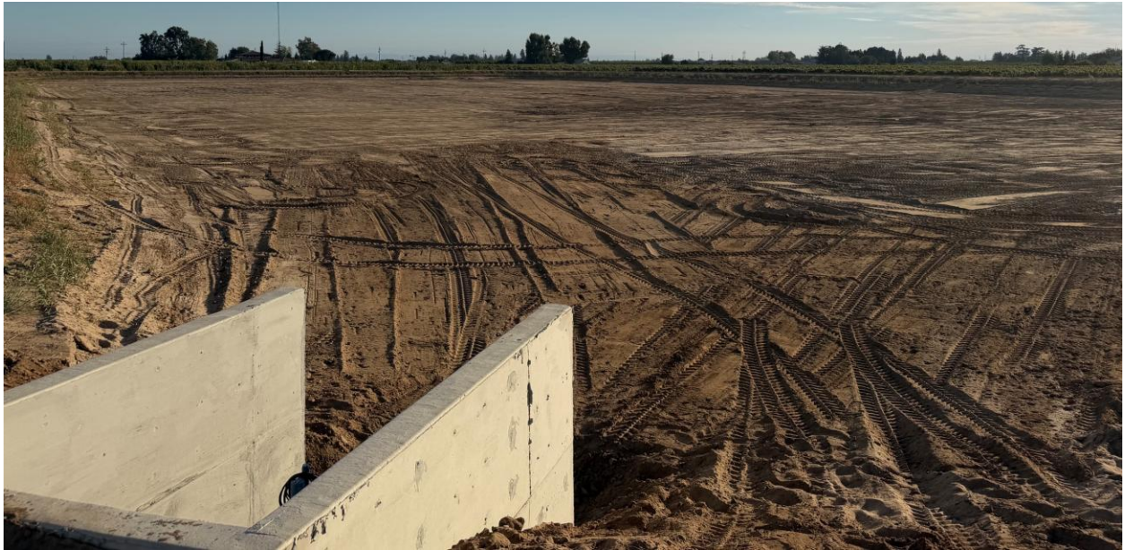
Teck Basin with the silt windrows all removed
