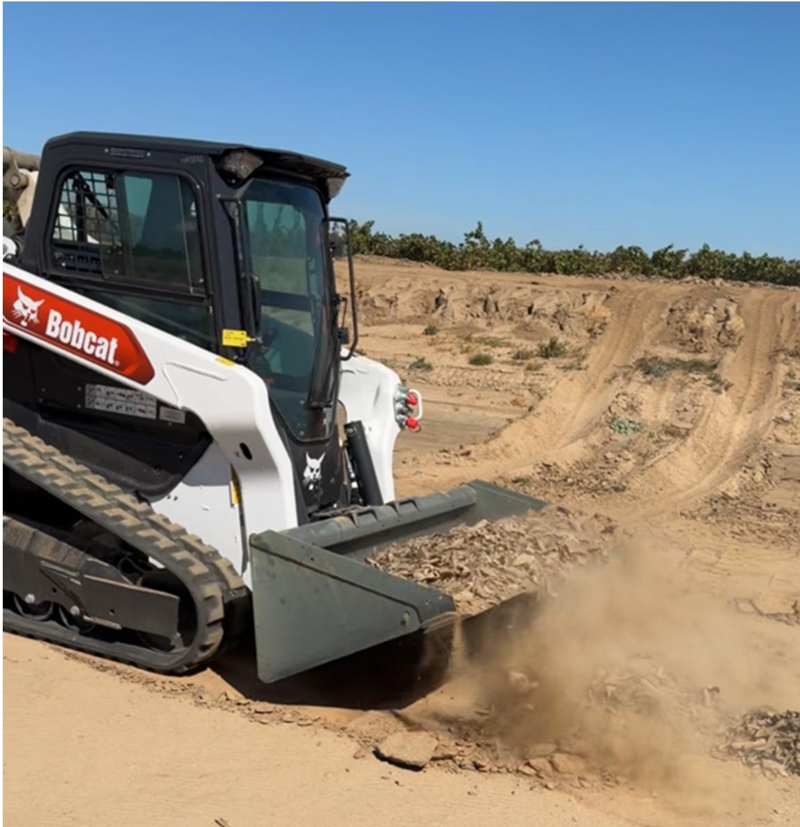
Silt Removal with the new Bobcat
